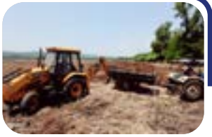
Disilting of Kharland Canal, Yashwantkhar Village, Roha, Raigad.
