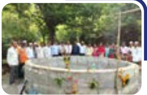
Rejuvenation of Well, Kadvad, Chiplun Taluka, Ratnagiri.
