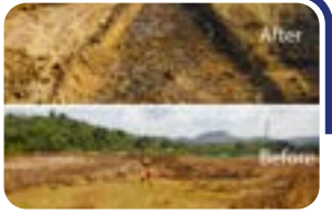
Yashwantkhar Village Excavation Work, Roha, Raigad.
